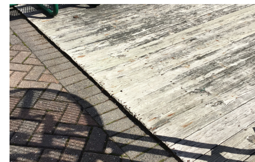
Fig 033. Uneven Pavement Exceeding 1/2"
