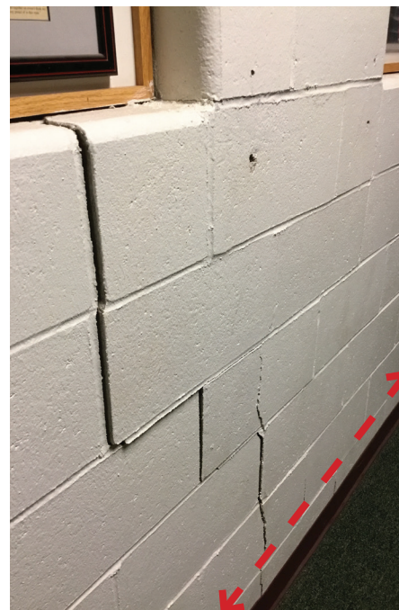
Fig 039. CMU Wall Shifted Out Of Plumb
