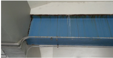
Fig. 045. Tower Ramps - Steel Beam Corrosion
