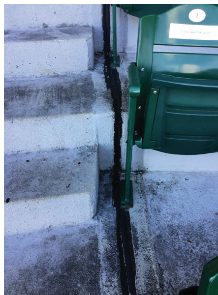
Fig. 102. Seating Straddling Expansion Joint
