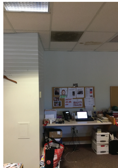
Fig. 128. Stained Ceiling Tile In Admin. Space
