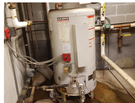
Fig. 063. Boiler Scheduled For Replacement - Much Sooner Than Typical (6 Years Old)
