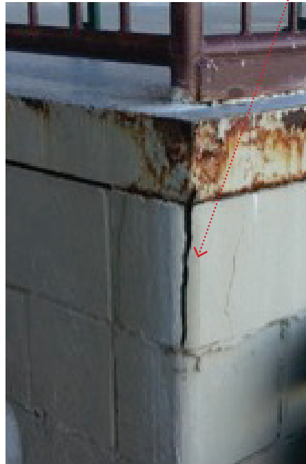
Fig. 047. Corrosion Due To Water Infiltration
