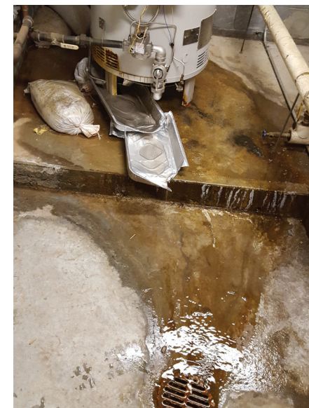
Fig. 055. Actively Leaking Domestic Hot Water Heater
