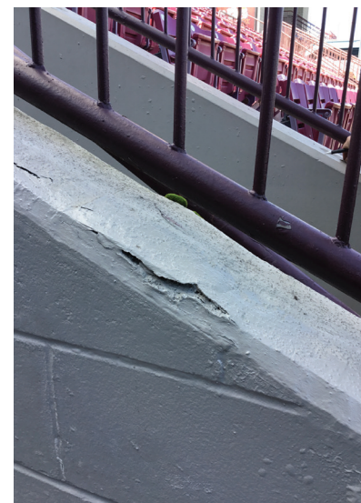
Fig. 110. Moss Growing Due to Standing Water
