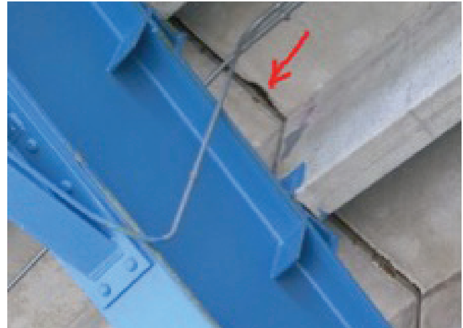
Fig. 049. Shims Involuntarily Moving
