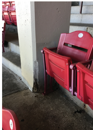
Fig 107. Major Chips & Cracks At Columns
