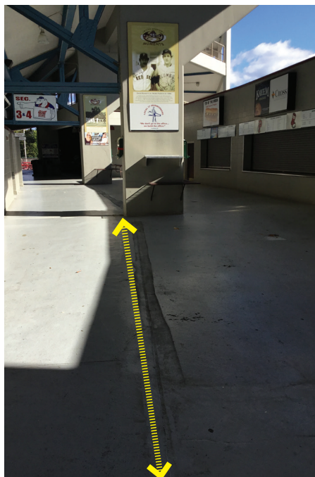
Fig 037. Sample Construction Joint
