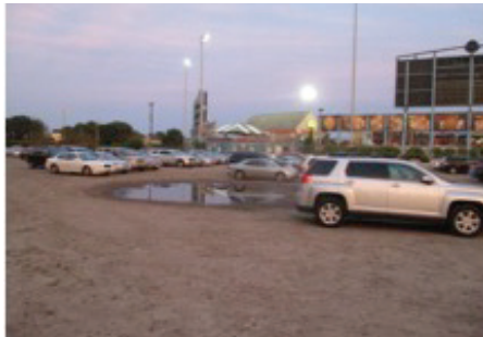
Fig. 020. Example of Ponding Water
