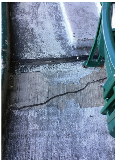
Fig. 104. Major Cracks In Horizontal Assembly
