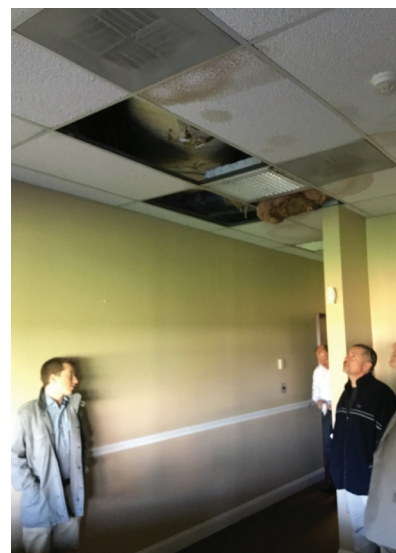
Fig. 108. Major Water Damage At Suites
