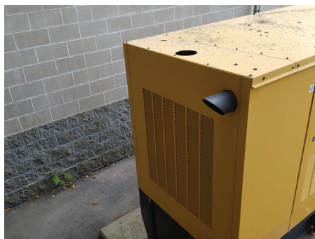
Fig 058. Generator Exhaust To Be Extended To Roof
