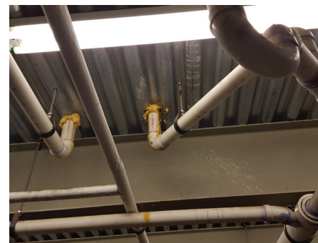
Fig. 062. Areas Of Water Infiltration @ Deck Drains
