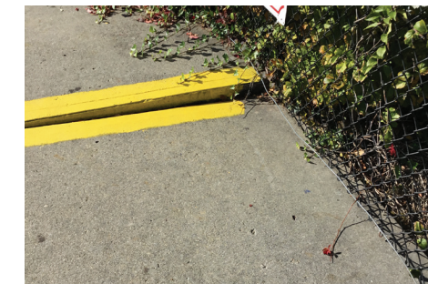
Fig 027. Example of Pavement Differential Settlement
