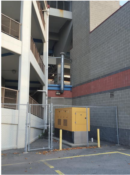
Fig. 056. Domestic Hot Water Heater Vent Termination Below Roof And Above Walkway - Note Proximity To Generator
