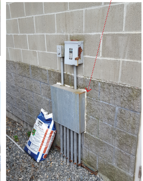
Fig. 074. Exposed Electrical Switching
