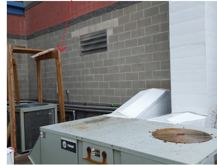
Fig. 070. Example Of At Grade HVAC Unit
