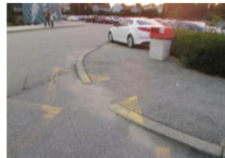
Fig 026. Example of Missing/Deteriorated Striping
