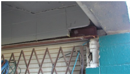
Fig. 046. Failing Lintel Support
