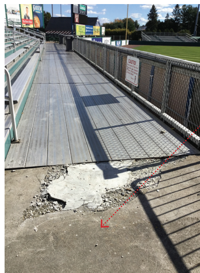
Fig. 031. Bleacher Construction Joint
