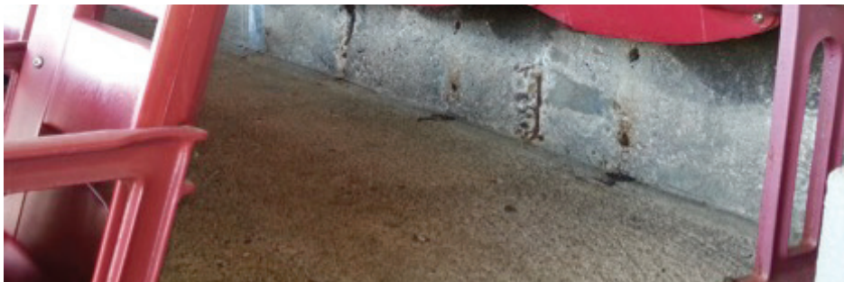
Fig. 048. Exposed Rebar - Rust/Corrosion
