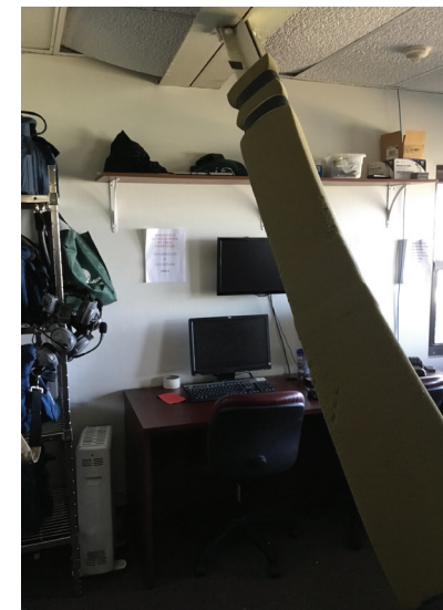
Fig. 130. Head-Knock Condition @ Press Box
