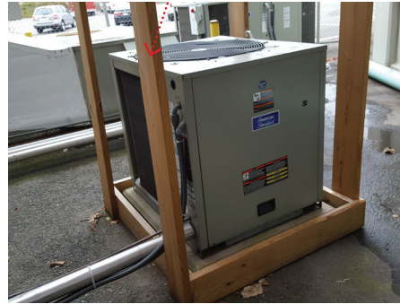
Fig. 067. Example Of At Grade HVAC Unit
