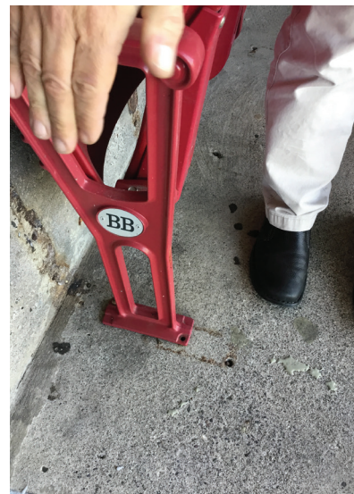
Fig. 109. Missing Fixed Seating Hardware
