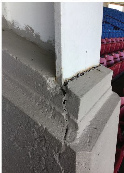
Fig. 105. Cracked Concrete = Water Entry
