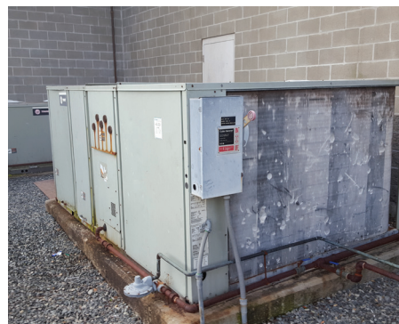
Fig. 053. 1998 Vintage On-Grade AHU - Damaged Coils & Corrosion - Note Pressure Relief Vents & Gas Regulators
