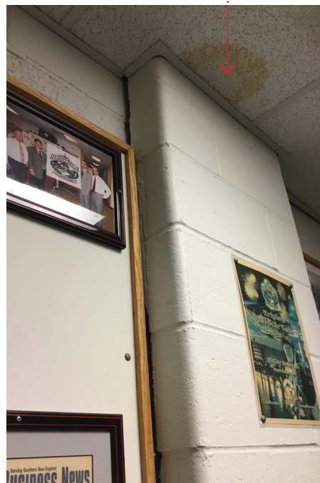
Fig 038. Example Of CMU Wall Movement
